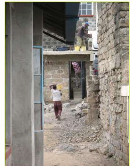
Community workers building new homes
